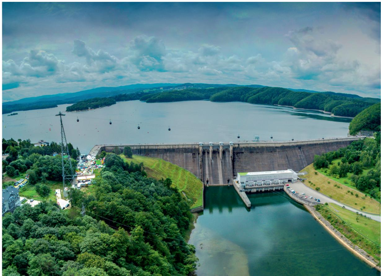
The water dam in Solina is the largest dam in Poland, and its height reaches 81,1 m, length 664,8 m, and width at the crown is 8,8 m.
